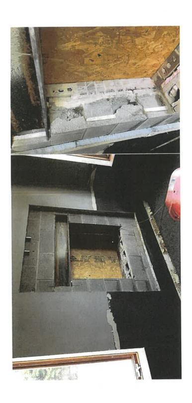
In cases where the baby box is installed in a structural wall, a support beam may need to be installed. Please note: These pictures were taken before the wood frame was installed. Above are examples of a location where a steel beam has been installed.
